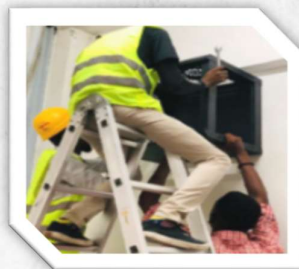
Network Cabinets Installation
